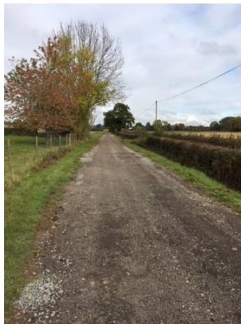
Photo of access track taken just north-east of application site, looking north towards A417
