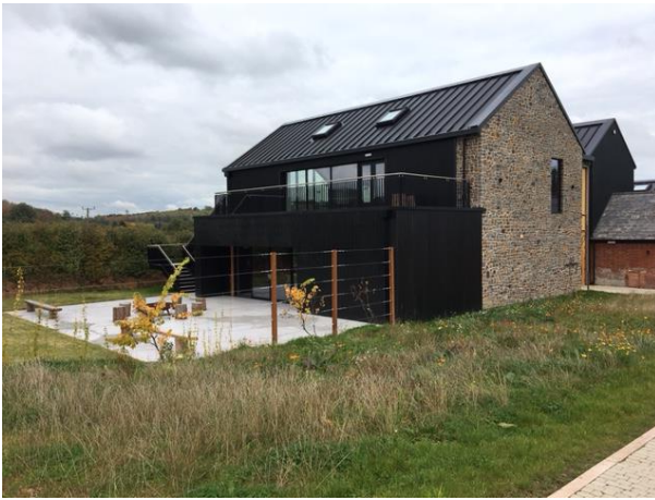
South-west elevation looking at balcony
