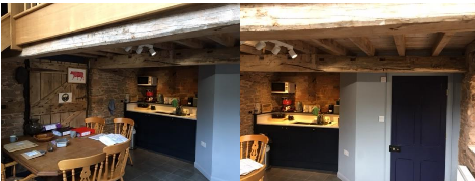
Ground floor of Barn
