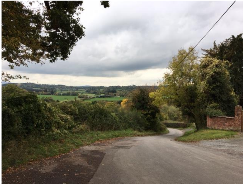
Photograph taken on U65030 adjacent Redhill looking southbound towards Crumplebury
