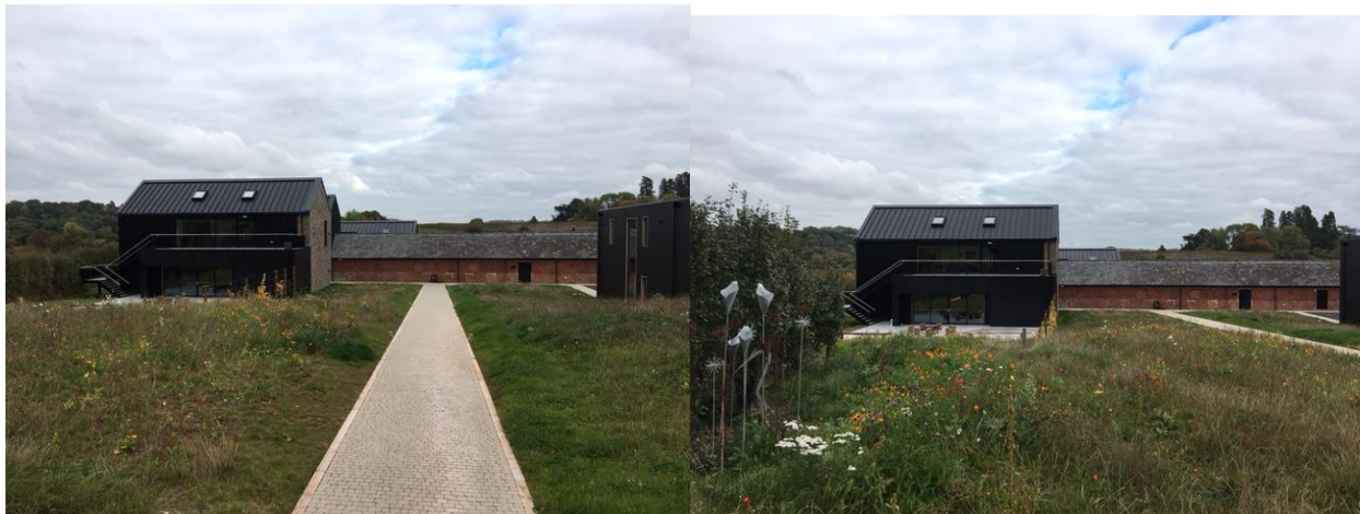
West elevation looking towards main buildings
