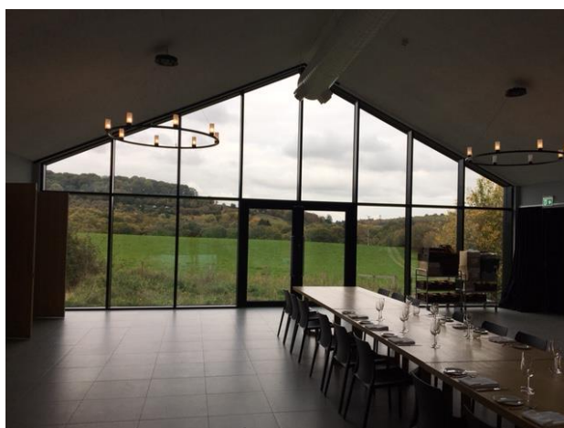
Photograph taken within Great Hall, looking towards Badley Wood Common, noting fixings to accommodate acoustic curtain
