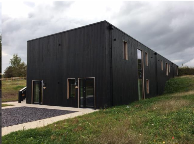
North-west elevation looking to accommodation
